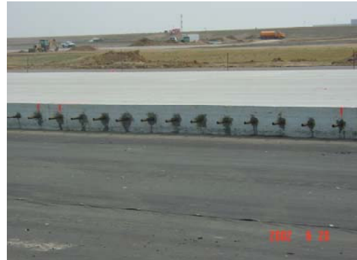
Figure 8.4 – Dowel bar installation along a longitudinal construction joint
